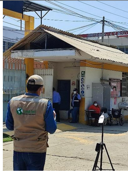
FOTO 19: PM-018: Puerta principal del hospital 13:50:08 horas
